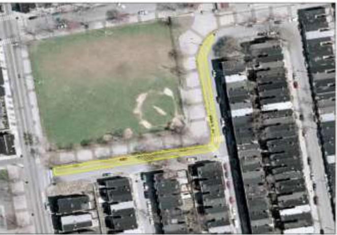
Street Tree Trenches
