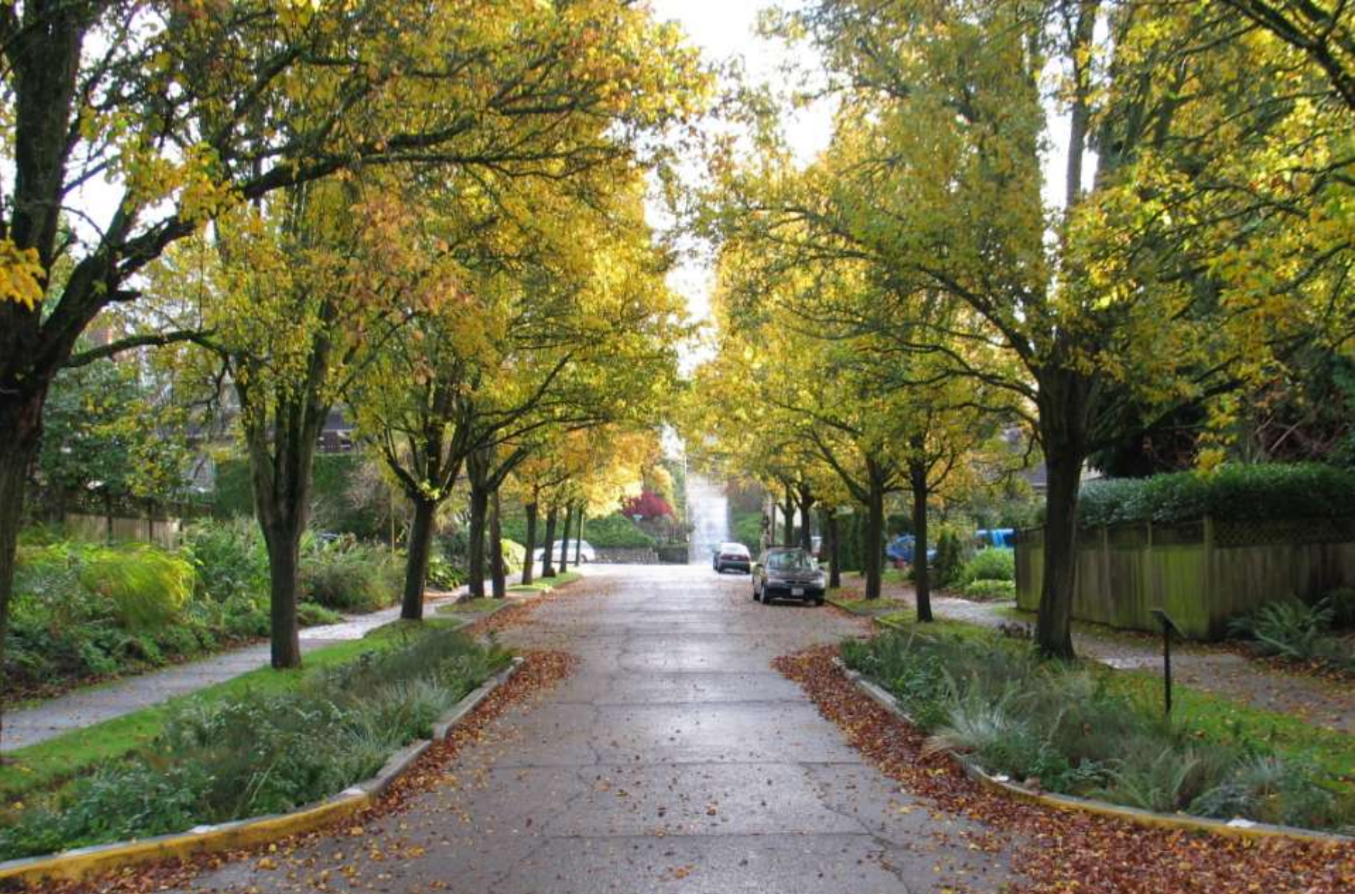
NE Siskiyou Green Street – Stormwater Curb Extensions
